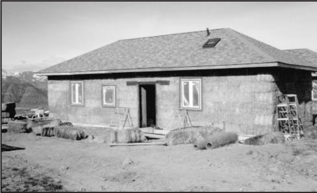
A straw bale house taking shape
